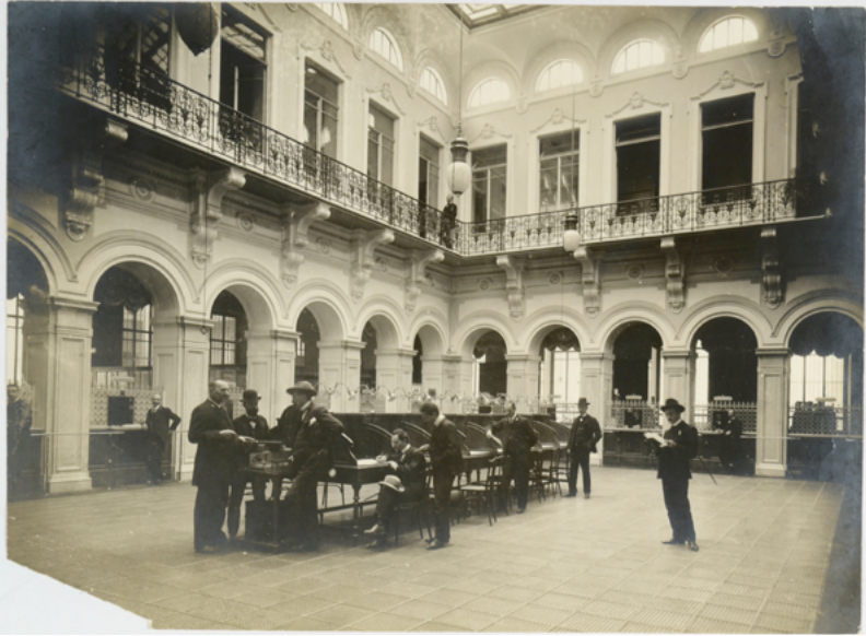
Fig 3. Headquarters of Istituto delle Opere Pie di San Paolo in Turin in via Monte di Pietà. Ground floor hall, home to lending and treasury activities, Turin, early 20th century.
