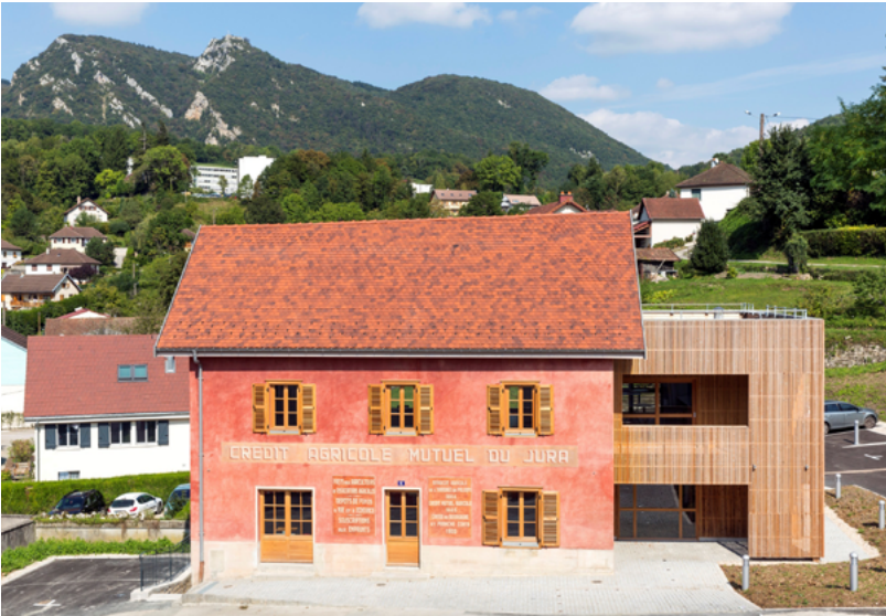
Figure 3: The office of the Maison de Salins Foundation in the restored building of the first local bank in Salins-les-Bains.
